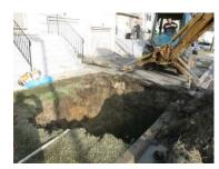
Concrete injection company drilled a hole through the 4" water main servicing water to the building from the city. The break showed to be directly underneath fiber optic cables and was inaccessible with excavation equipment.
